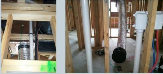
Photo 1 – Duct blaster connected to main trunk line before the air handler is installed
